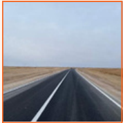
Infrastructural development program
